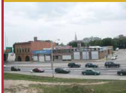
The site of MICA's proposed project is at the intersection of Mount Royal and North Avenues in Baltimore.
