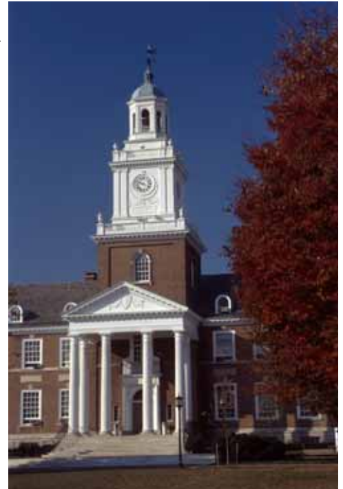
Gilman Hall, built in 1915, is the flagship structure of Johns Hopkins' Homewood campus.
